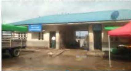
MPA Port Office + Police Station
