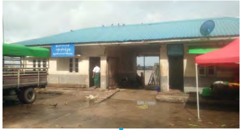
MPA Port Office + Police Station
